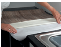
3. Peel off 10 cm of the paper from the film.
