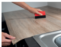
4. Apply the film and press it down with the squeegee.
