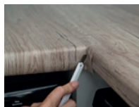
5. Cut or trim the film with the cutter.
